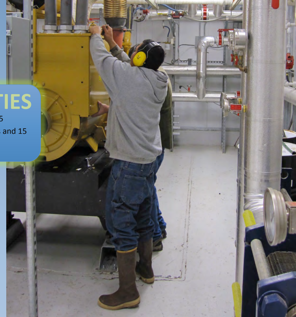
Angoon power house operator training on new power house module during construction
